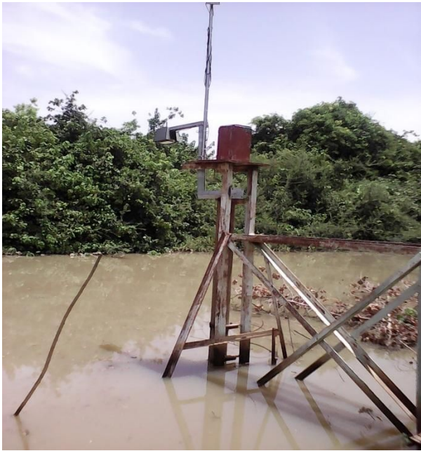
a) Cat-walk before installation of the device
